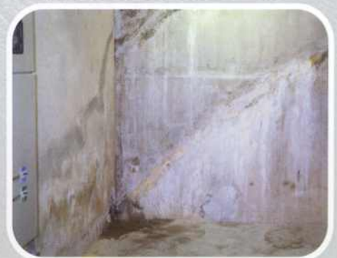
CRACK REPAIR DAY SEVEN
