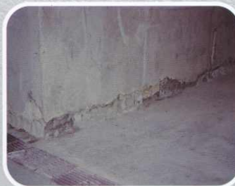
COLD JOINT REPAIR — AFTER
