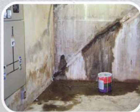
CRACK REPAIR DAY TWO
