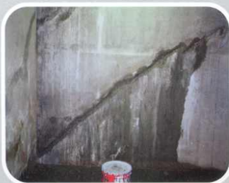
CRACK REPAIR DAY ONE
